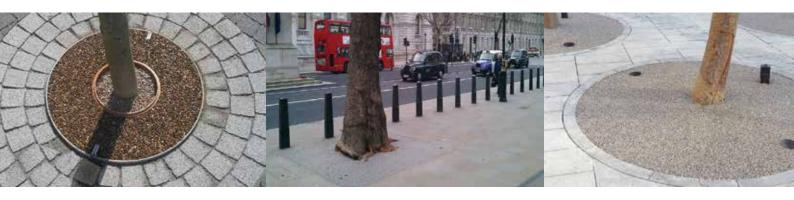
Addagrip TP Resin is normally mixed with a 6-10mm grade of washed, clean and dry aggregate, and laid to create a porous surface. It is ideal for tree pits and light use footpaths.
