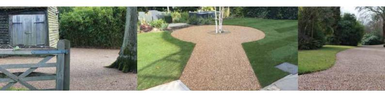
Addagrip Amber is a Resin Bound Surfacing System based on a blend of natural aggregates and a natural oil Aromatic Polyurethane resin where the colour is enhanced in the initial curing process.
